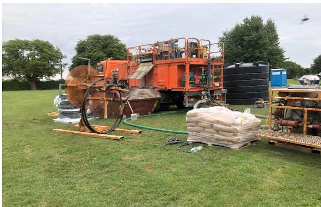
the school playing field where a new £750,000 automated boring machine, along with associated equipment drilled 10 boreholes to a depth of 96 meters and threaded in the flow and return pipes to extract the heat from the underlying rocks. In this case it was a thick layer of mudstone sandwiched between 2 bands of limestone. These outside works have been completed and the internal works are planned for half-term.
